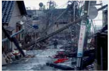
p.6 2024 Noto Earthquake
